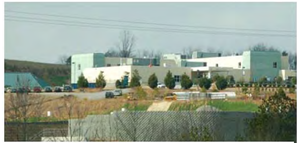
Piedmont Mountainside Hospital
