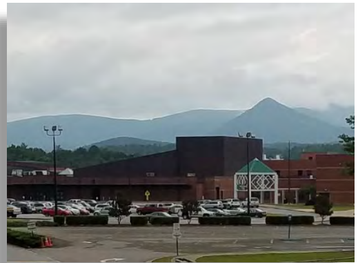
Figure 35: Pickens County High School
