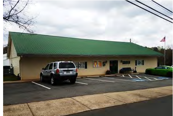
Figure 73: Nelson City Hall along Kennesaw Avenue
