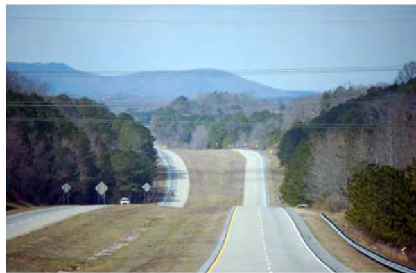
Looking north on Hwy. 515
