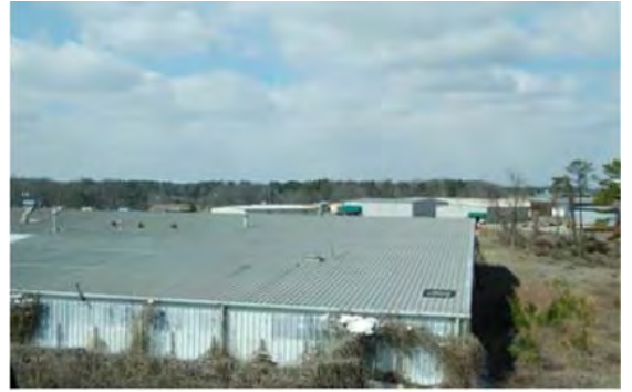
Figure 62: Typical industrial Structure located in Pioneer Industrial Park.
