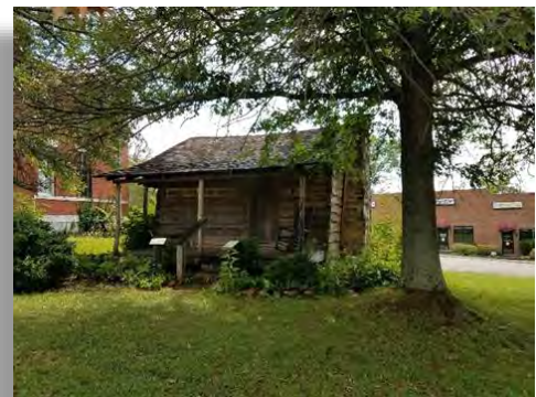
Figure 20: Historic Kirby-Quinton Cabin restored and relocated to downtown Jasper
