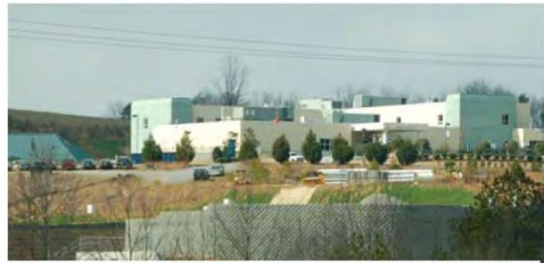
Piedmont Mountainside Hospital
